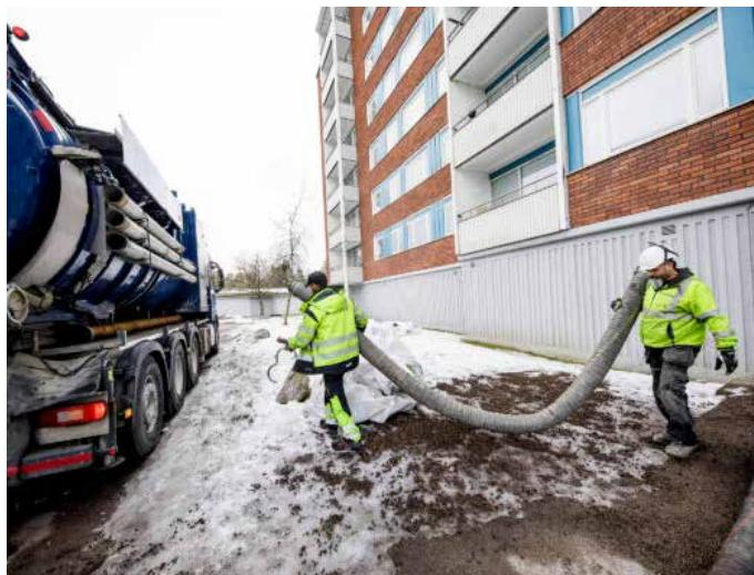
**DISAB Centurion™ LN30 is a truck mounted unit that can convey material using airstreams (pneumatic transport), created by either vacuum or overpressure.**
